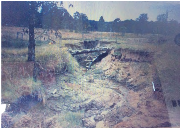
Erosion blow out prompting serious rehabilitation strategy
