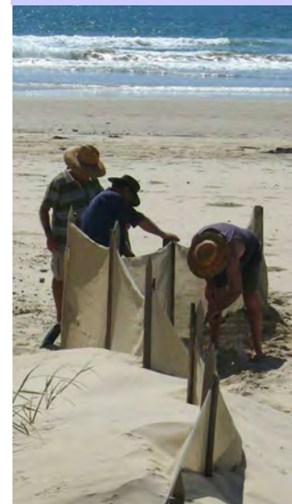
Construction of sand trap to prevent wind erosion and to enable Lake Cakora berm to rebuild
