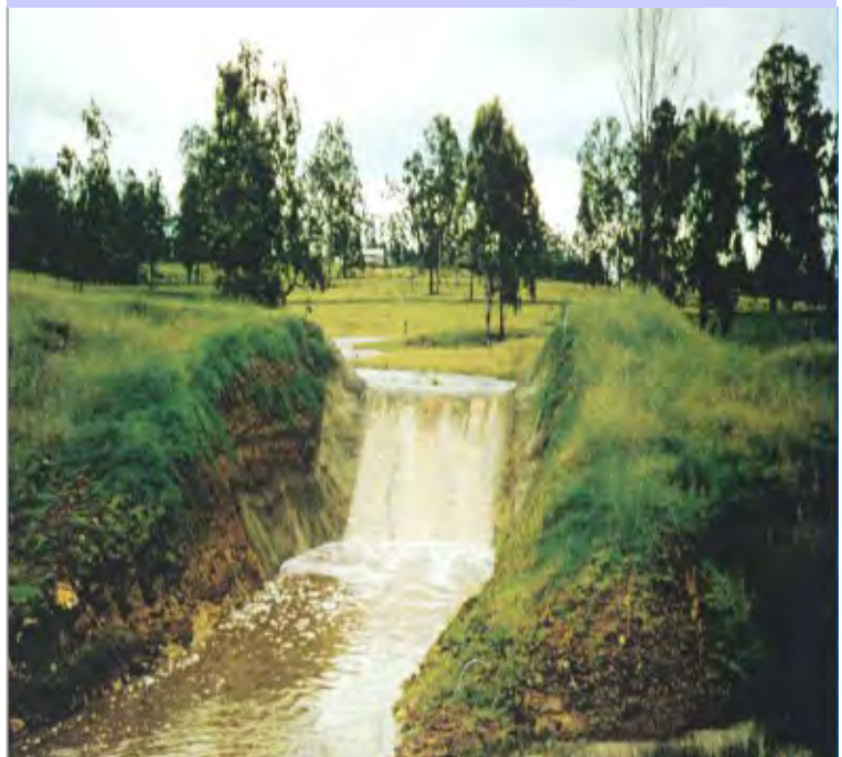
The rehabilitated area withstanding flood
