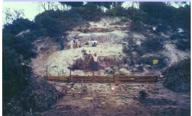
1995. Spooky Beach erosion control work in progress
