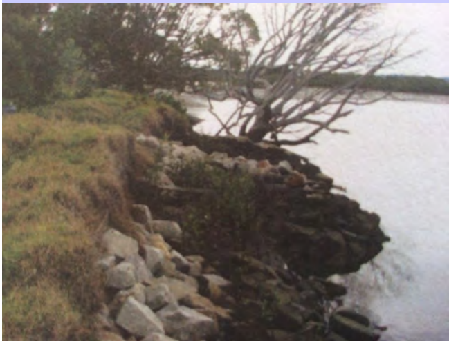
Solution: bank stabilised with rock fillets with mangroves recolonising and creating fish habitat
